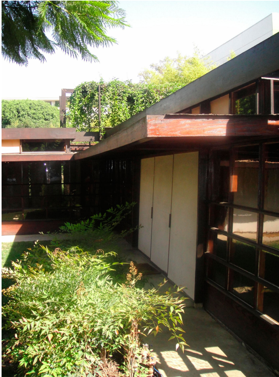
Figure 6. Clerestory window over a deep overhanging eave placed along the façade, Schindler House, Los Angeles.
