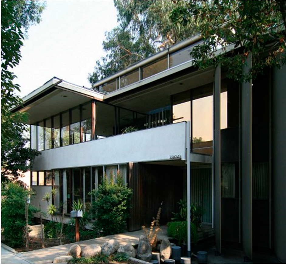
Figure 12. View of vertical louvers at VDL2 House, Richard Neutra. Located in Silver Lake, Los Angeles.
