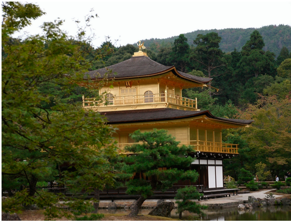
Figure 1. The temple of Kinkaku (Golden Pavilion) in Kyoto. Reflection in the water from gilded panels.
